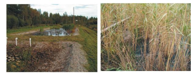
Figure 17. Sludge drainage beds are a well-proved method for sewage sludge management. With the planting of plants (e.g. common reed) a valuable humus soil is produced.
