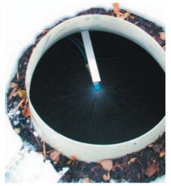
Figure 14. Spraying techniques improve soil filter techniques by efficient distribution and aeration or anaerobic water from sulphur hydrogen. A technique developed in Norway uses turbulent chambers spraying with 5-6 mm orifices. The nozzles can be installed in domes (like in the picture) or in a simple greenhouse or similar. Picture from Ångersjön, Hudiksvall, Sweden (photo P. Ridderstolpe).
