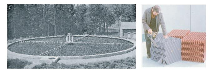
Figure 16. The trickling filter is a well-proved and robust technique for biological treatment of BODpolluted water. Earlier applications used stones but today plastic media is more common. (Photos: left from Metcalf & Eddy (1989), right from P. Ridderstolpe )
