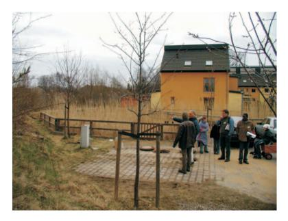
Figure 9. Vertical soil filter planted with common reed used for greywater treatment in an ecological residential area, Hamburg, Germany. The water is applied from the top and percolates vertically through the bed in an unsaturated flow. The dimensioned load is 60 l/m2/day ( photo: P. Ridderstolpe).
