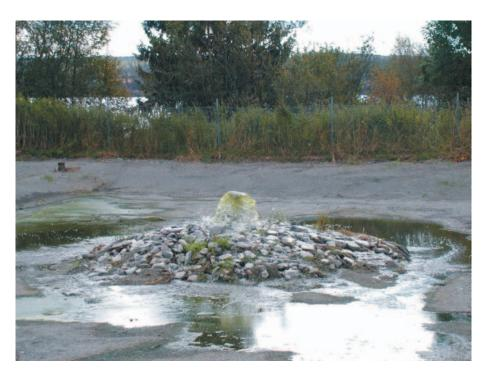
Figure 12. Open sand filter bed in Alsen, Krokom municipality in Sweden. Pre-treated wastewater is distributed on the surface by flooding (Photo: E. af Petersens).
